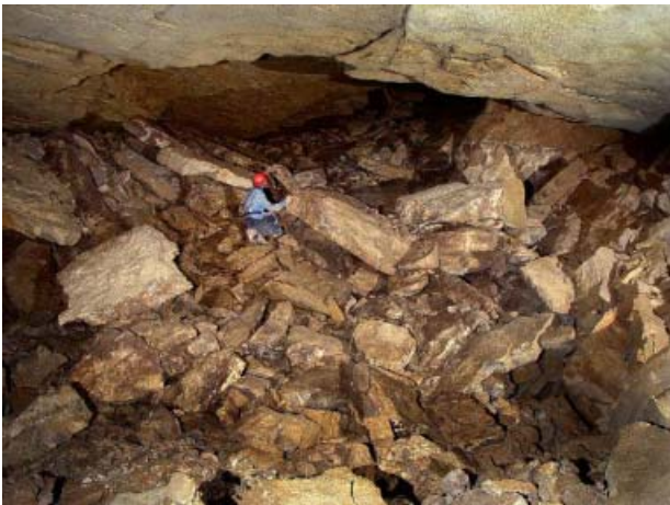
Fig. 10. Collapse at a passage intersection in Mammoth Cave, Kentucky. The strata are similar in age and character to those in Lost River Cave.
