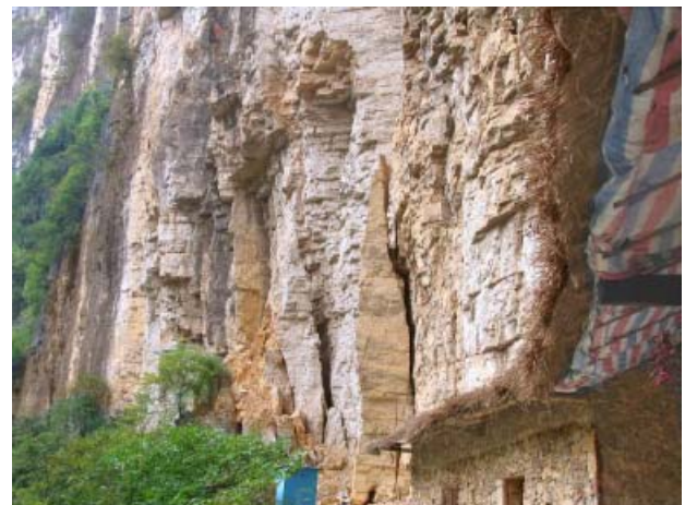
Fig. 7. Vertical fractures on the wall of Xiaozhai Tiankeng, Chongqing.
