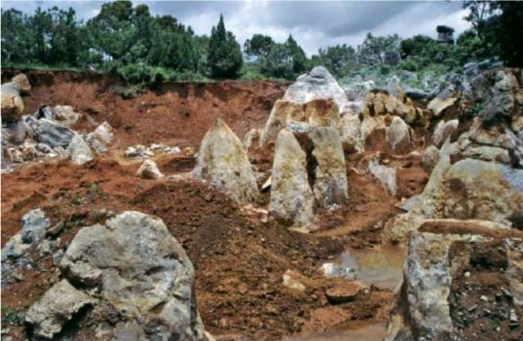
**Fig. 8.** Pinnacled rockhead partially exposed on a construction site in class kV ground at Lunan, in Yunnan, China. The original ground surface had only a few protruding pinnacle tips. Excavation to a lower level achieves a greater proportion of rock to soil for bearing purposes, but requires removal of the taller pinnacles.
